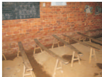
The current Shu An Church in Hubei province meets in a old grain storage facility with a leaky roof. Can you imagine sitting on these pews?
