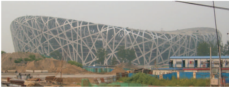
Beijing's New Olympic Stadium is already showing signs of environmental damage
